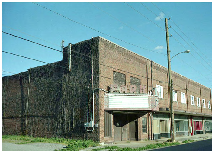
The Park Theater in Middlesboro, located in Bell County in the eastern part of Kentucky, was last in operation in the early 1980s. Credit: Jared Hamilton
