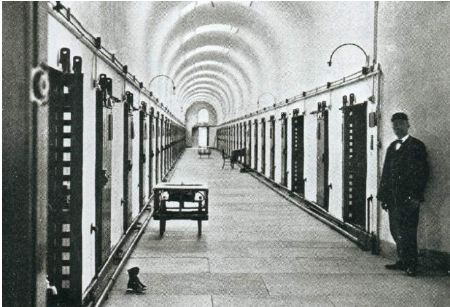
Eastern State Penitentiary, opened in 1829 on the Pennsylvania System (Photo courtesy Eastern State Penitentiary)
